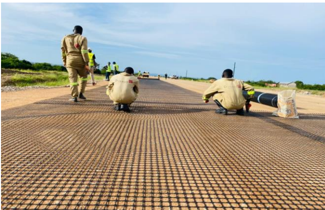
Installation of Geogrid Upper Subgrade Layer
