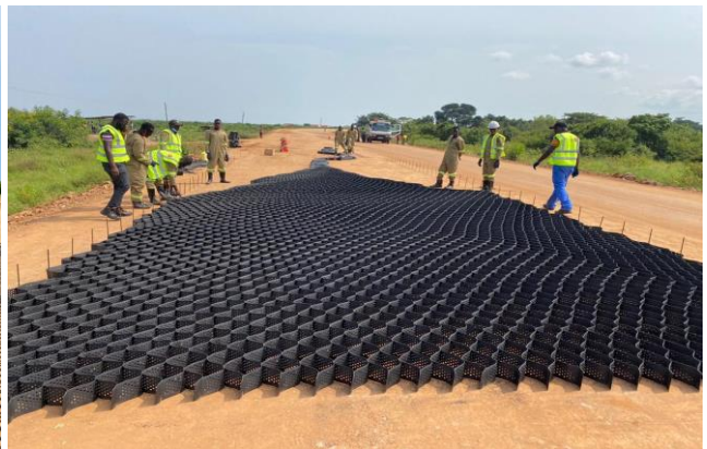
Installation of PRS Neoloy Geocell Sub Base Layer
