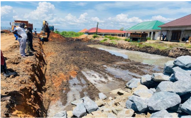
Existing Subgrade Condition
