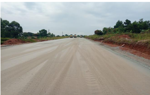
Finished & Compacted Base Layer
