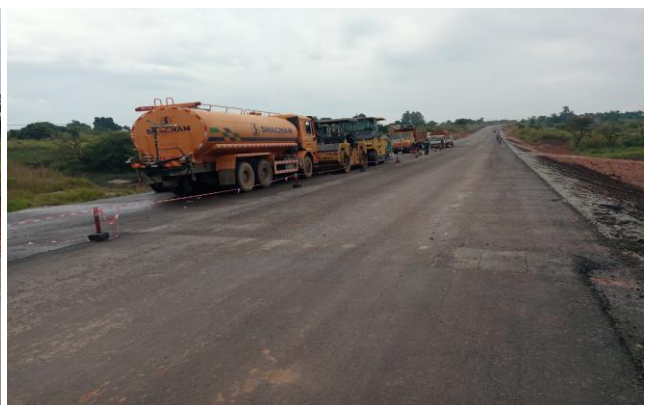
Installation of Final Asphalt Layer
