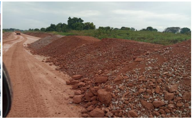
Pioneer Layer Preparation
